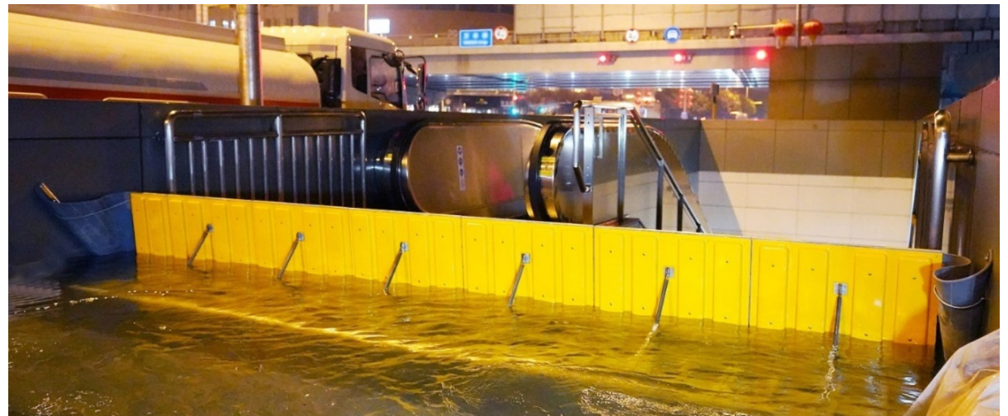
BJMTR pilots the installation of smart flood control baffles
