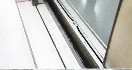
Screen doors of Line 4, Daxing Line, Line 14 and Line 16 are equipped with gap rubber and LED lighting post, effectively preventing passengers from being hurt by the screen doors.
