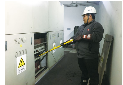
Working with the upgraded DC live-line tester
