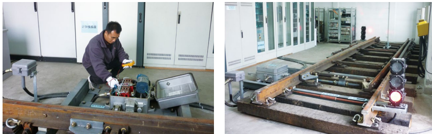
Training and testing base for Communication & Signaling Maintenance Department
