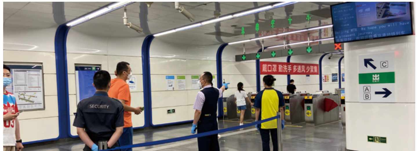
Fast access after replacing one-way AFC gates with two-way AFC gates in Jiangtai Station
